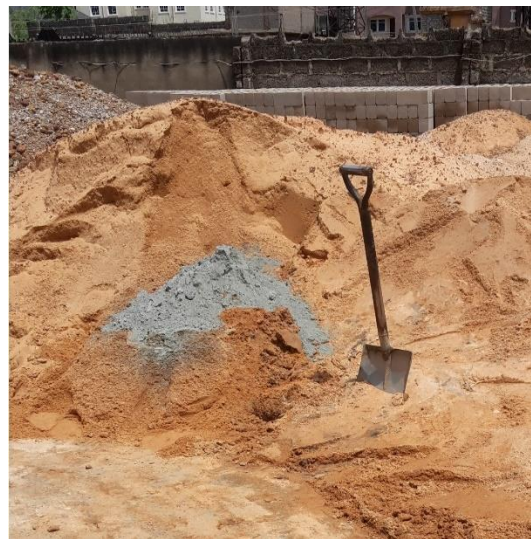
Fig. 3 Batching by Estimation/guesstimating quantities of cement, sand, and water at the site
